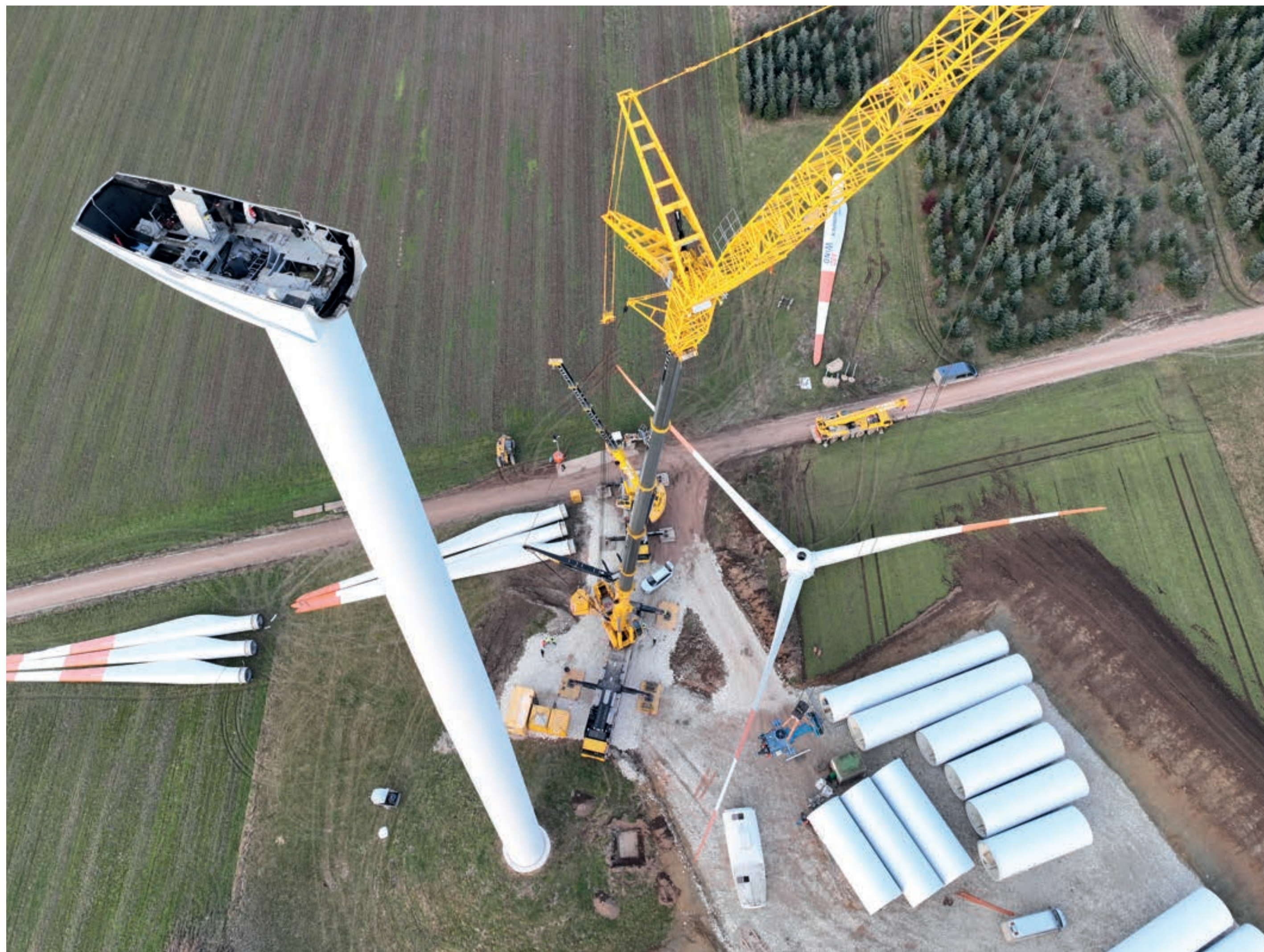
Dismantling wind farm
