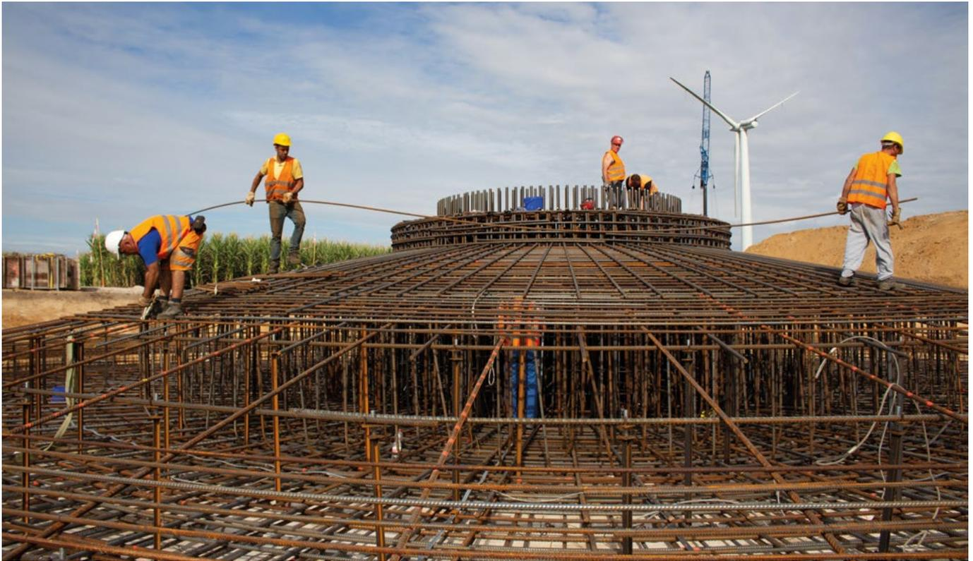
Construction of the foundation for the Wennerstorf wind farm in Germany: In this repowering project, four older turbines were replaced by two modern ones. With the two 4.5 megawatt Nordex N149 generators, the new wind farm produces three times as much electricity as its predecessor.
